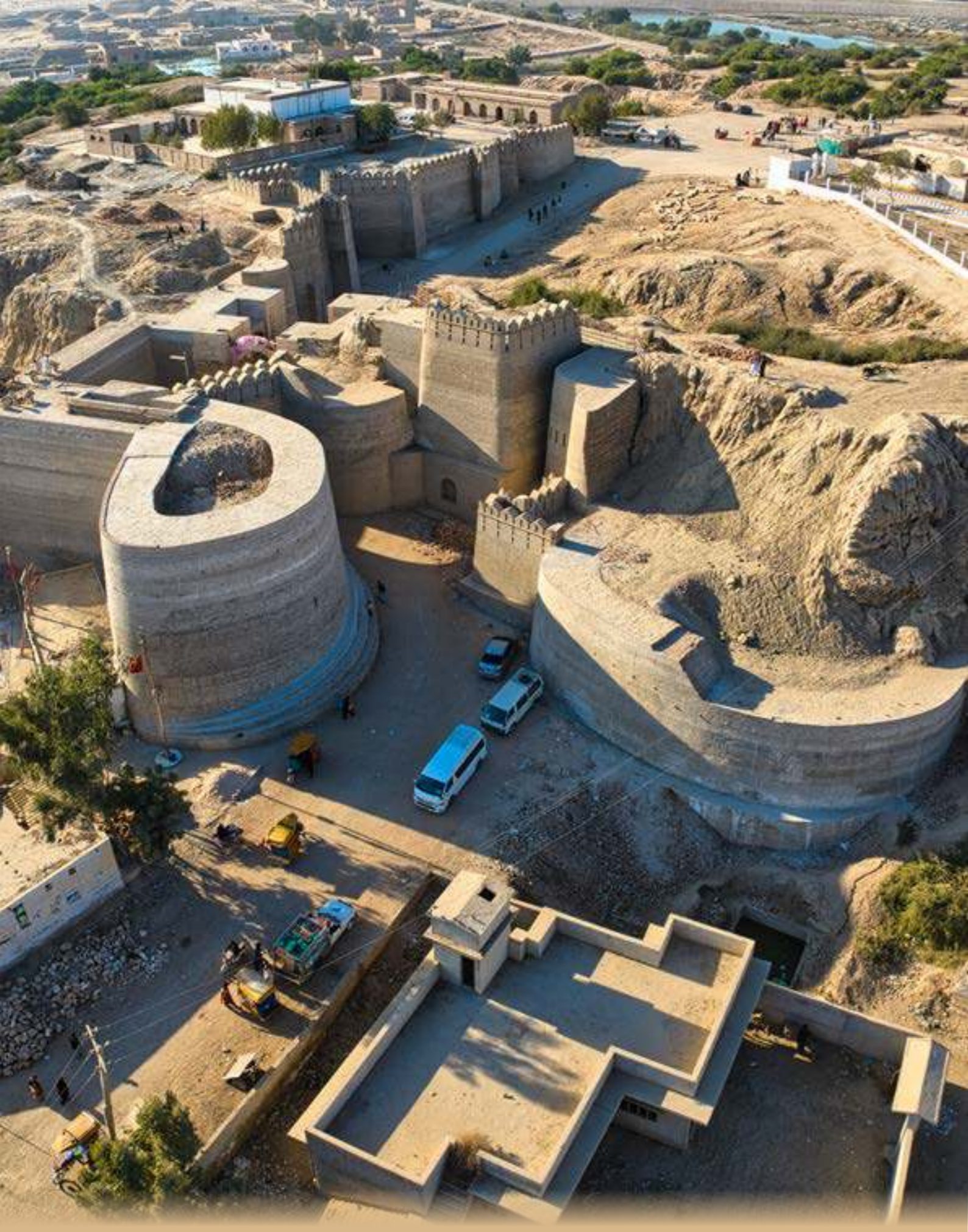
From the sky, brick by brick: The revival of Sehwan Fort
