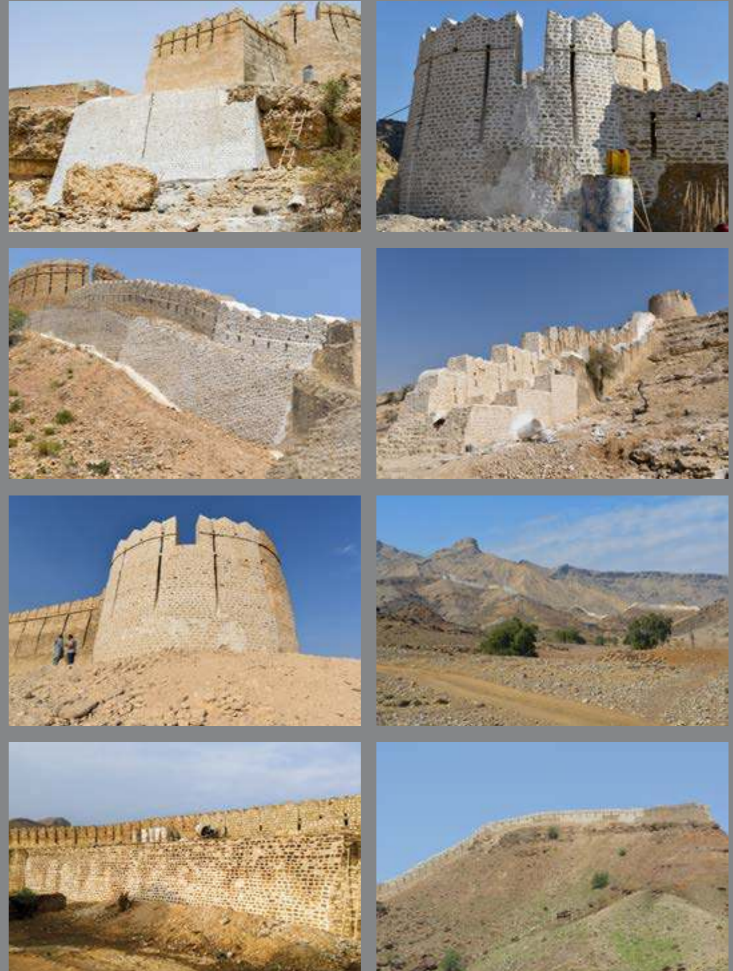
This series showcases the same locations following careful restoration work. The images document the revival of architectural elements, illustrating the results of the conservation efforts undertaken at the fort.
