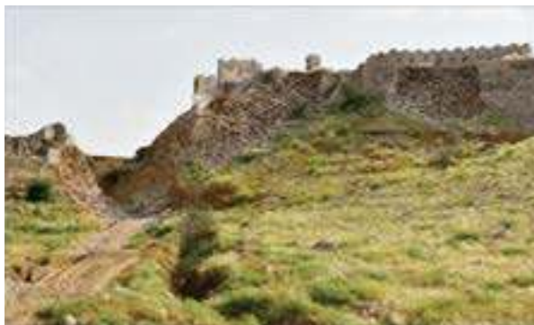
Rain damage at Shahper Gate and walls
