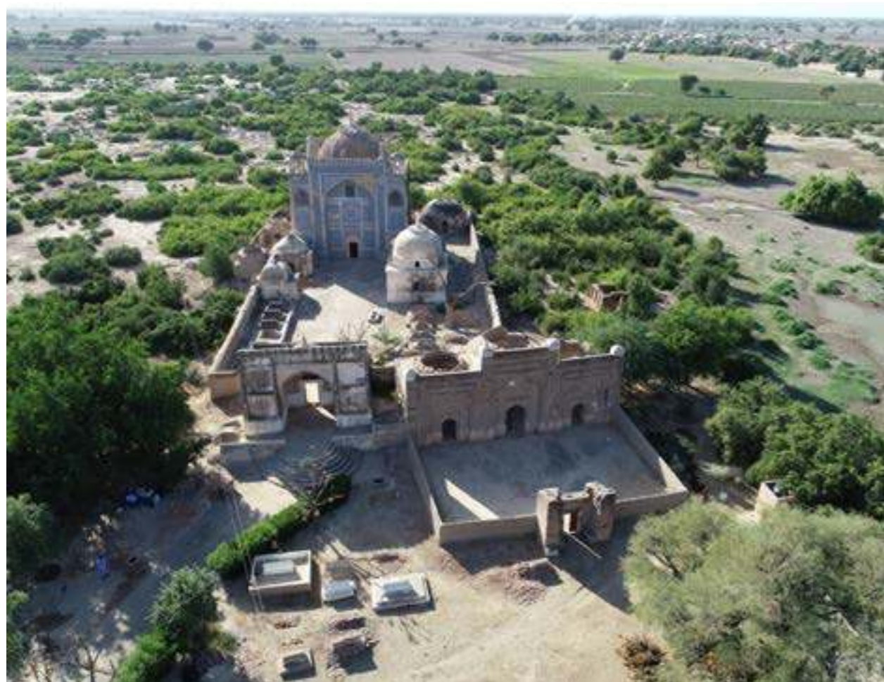
Rain damages at Mian Noor Muhammad Kalhoro, Dadu
