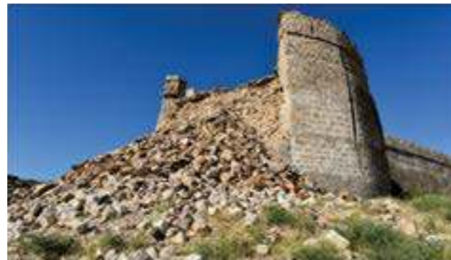
Bastion eroded at Meeri Fort, Ranikot
