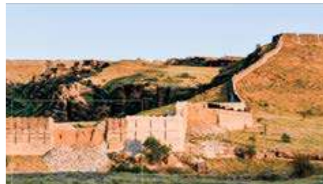
Rain damage at Mohan Gate, Ranikot
