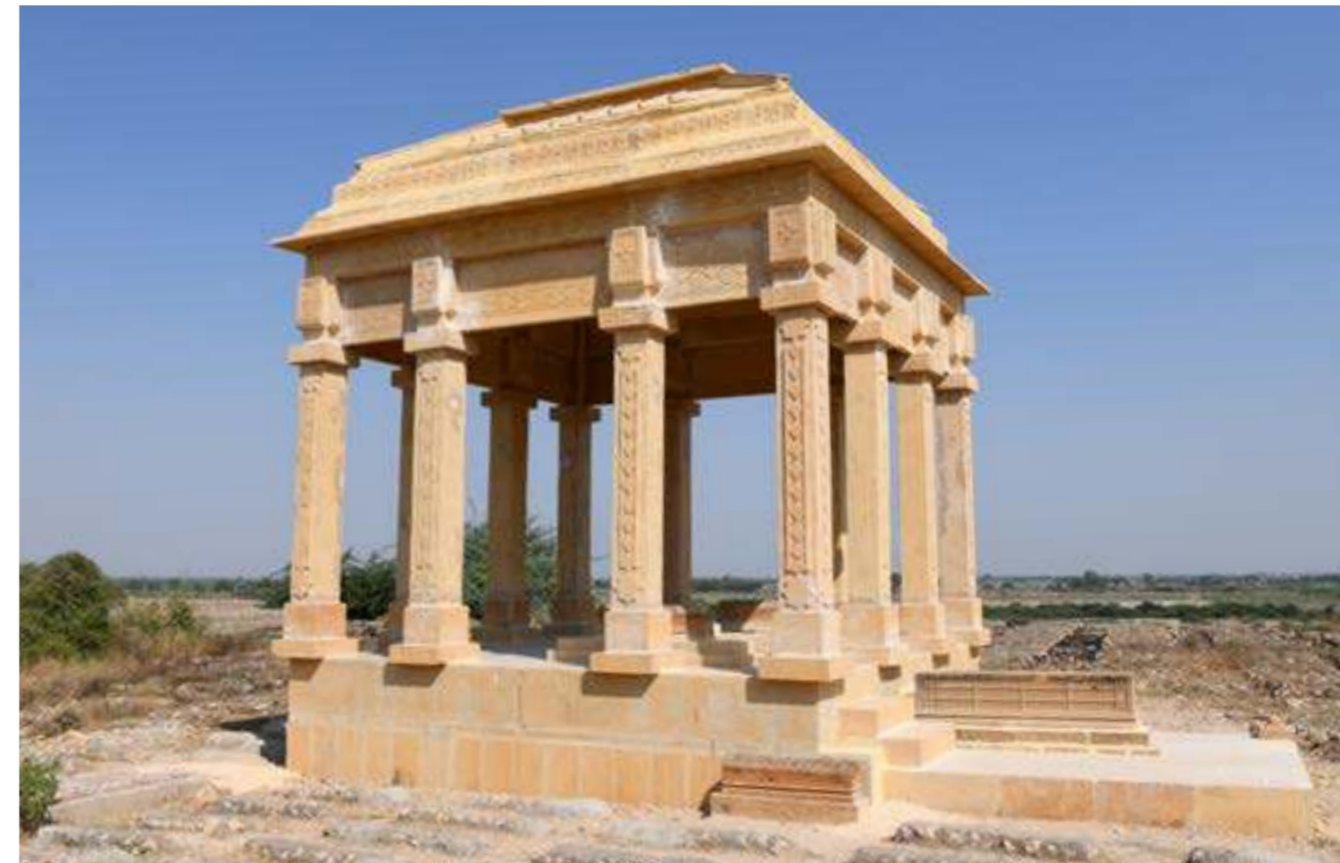
Rehabilitated Mir Ali Sher Qani's mausoleum
