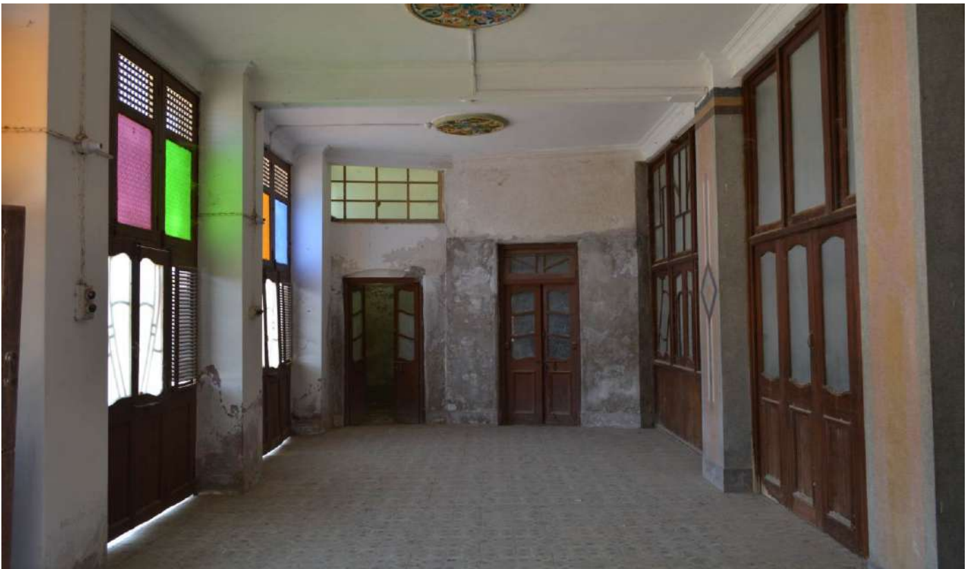
INTERIOR VIEW FRONT FIRST VERANDAH
