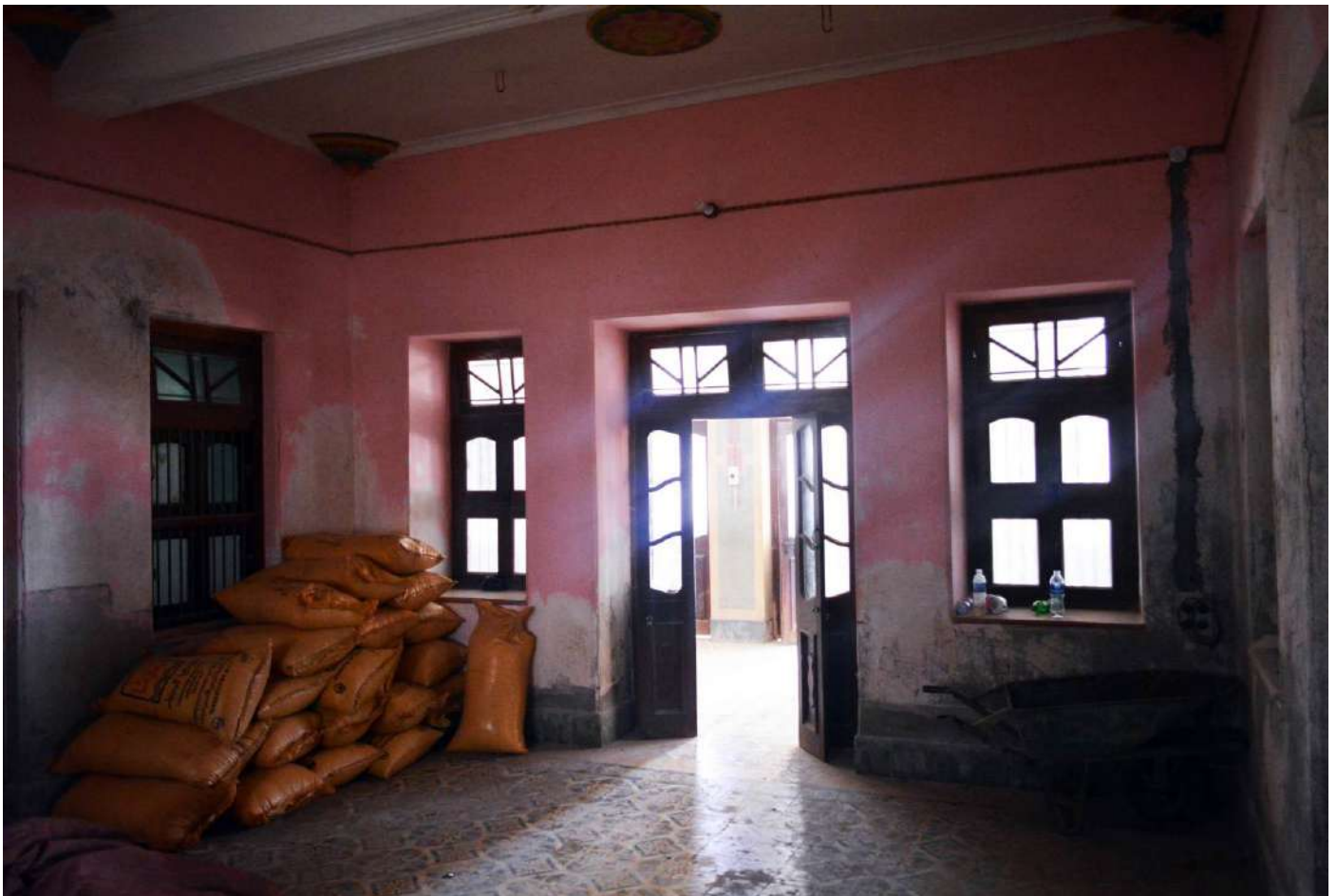
INTERIOR VIEW OF ROOM NO:2
