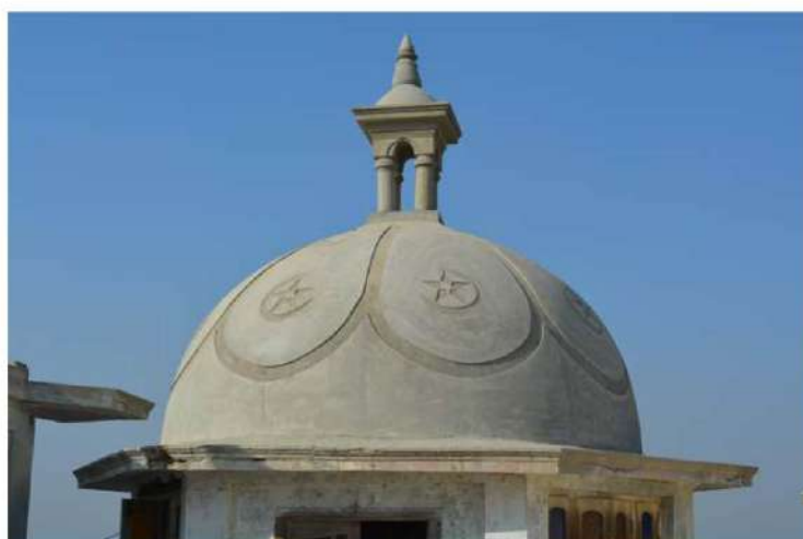
Northern (Backside) Dome Progress upto December 2016
