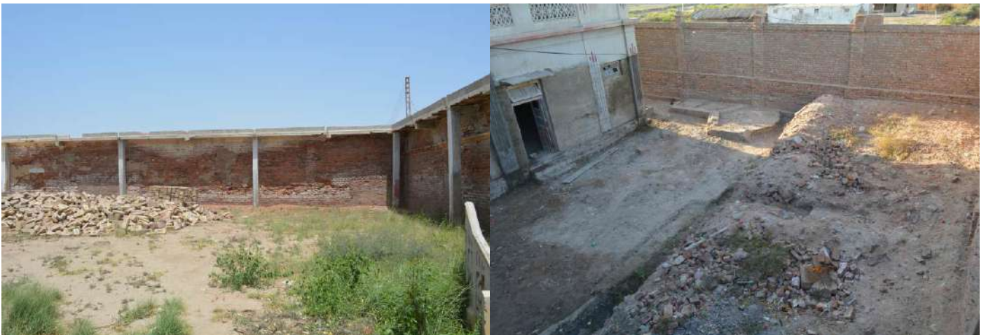
INTERIOR VIEW OF BOUNDARY WALL
