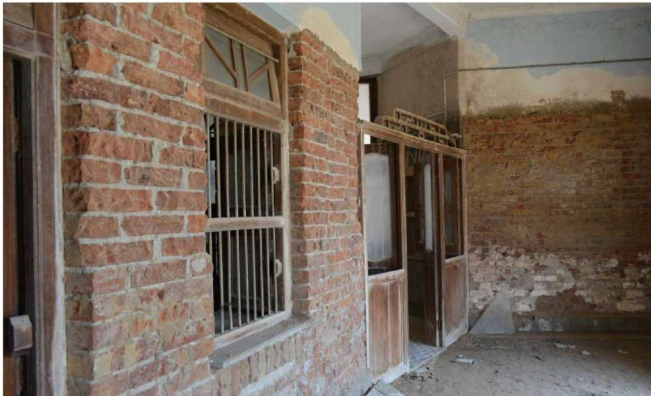
Removal of plaster upto lintel level
