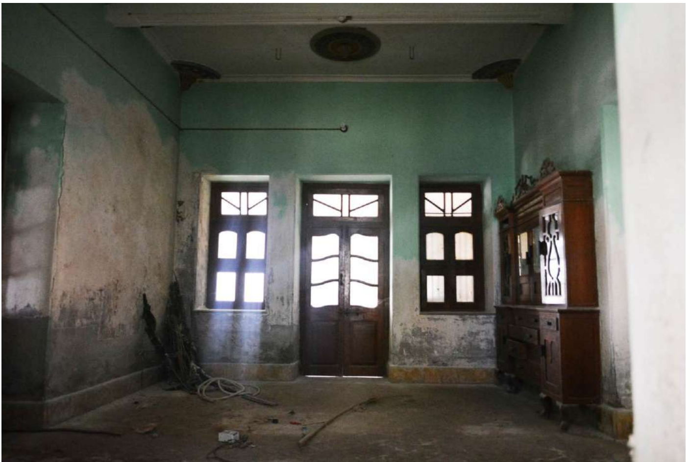
INTERIOR VIEW OF ROOM NO:3
