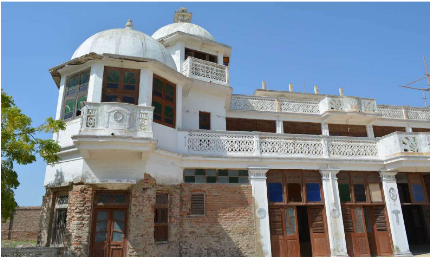
EXTERIOR VIEW OF BUILDING
