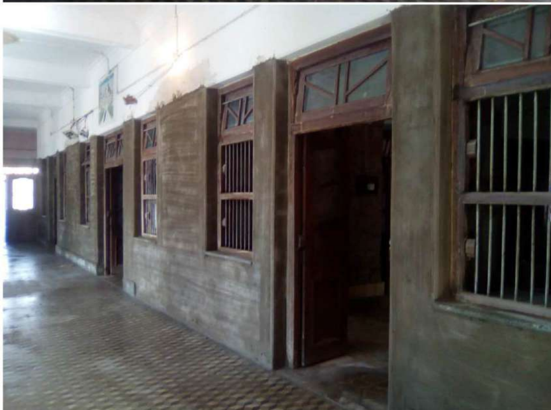
1st Coating of Cement
