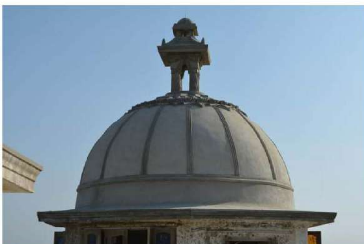
Northern (Backside) Dome Progress upto December 2016
