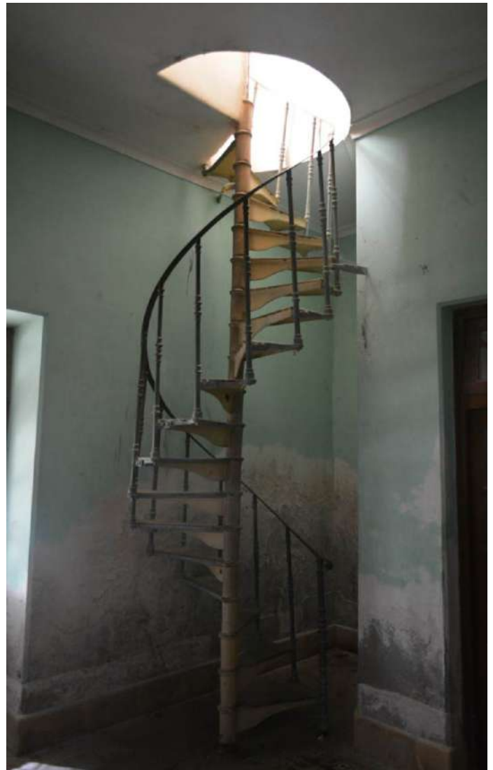
LEFT ROOM GROUND FLOOR
