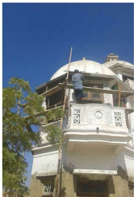
Mason working on Chhaja on the top floor
