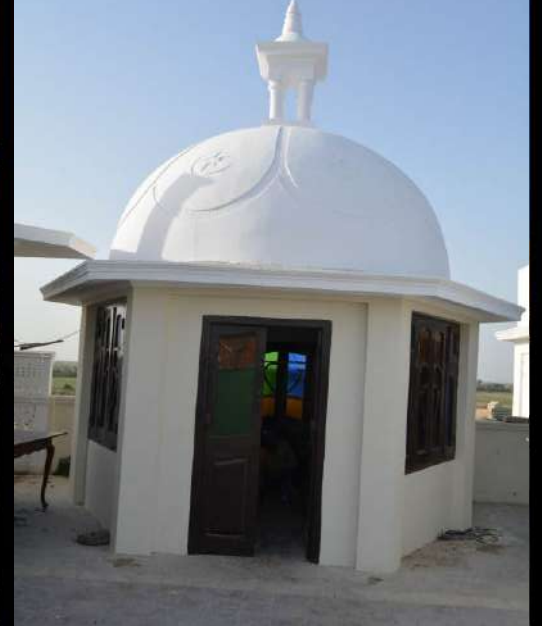
BACK SIDE DOME AFTER
