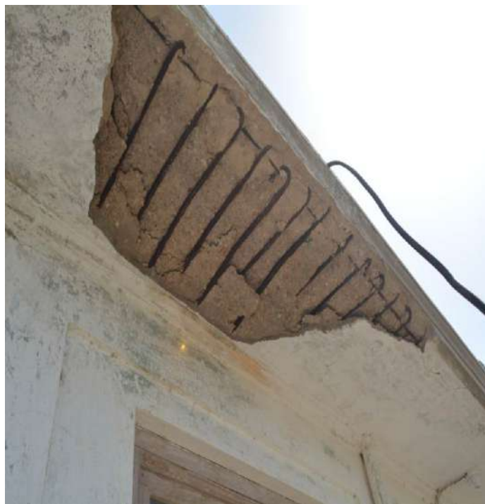
TOP ROOF SLAB
