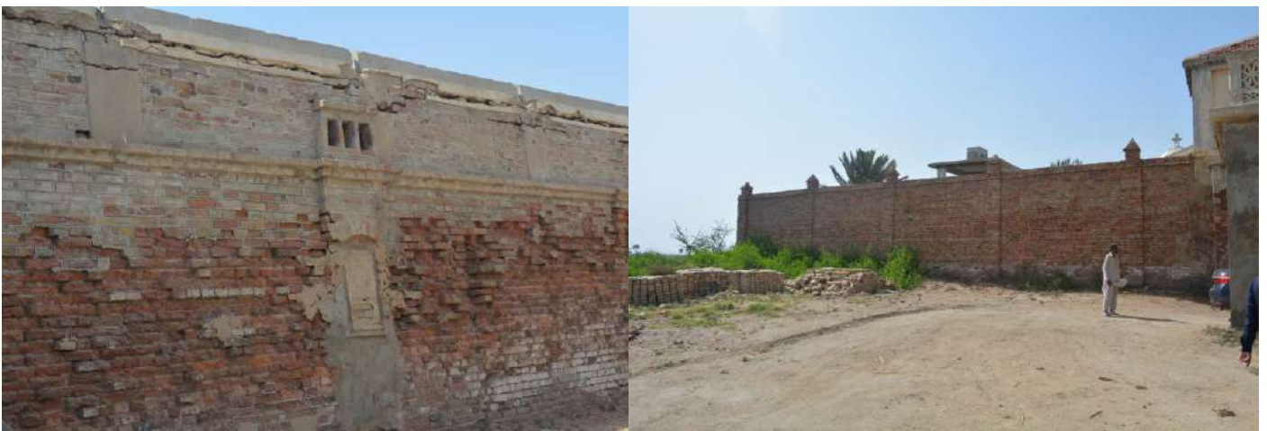
EXTERIOR VIEW OF BOUNDARY WALL
