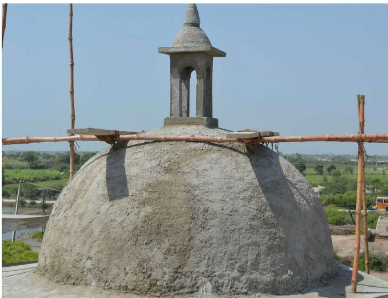
Progress upto September 2016
