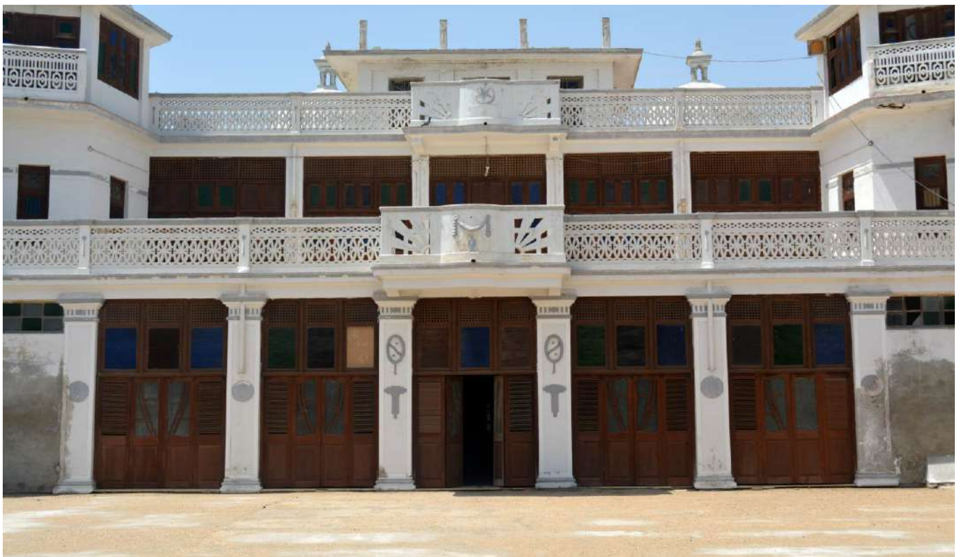
EXTERIOR VIEW OF GROUND FLOOR
