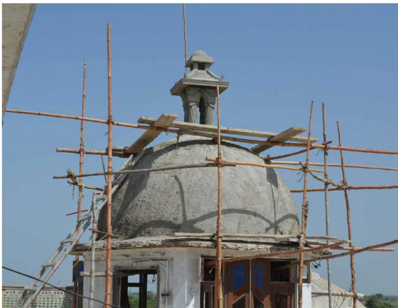
Progress upto September 2016
