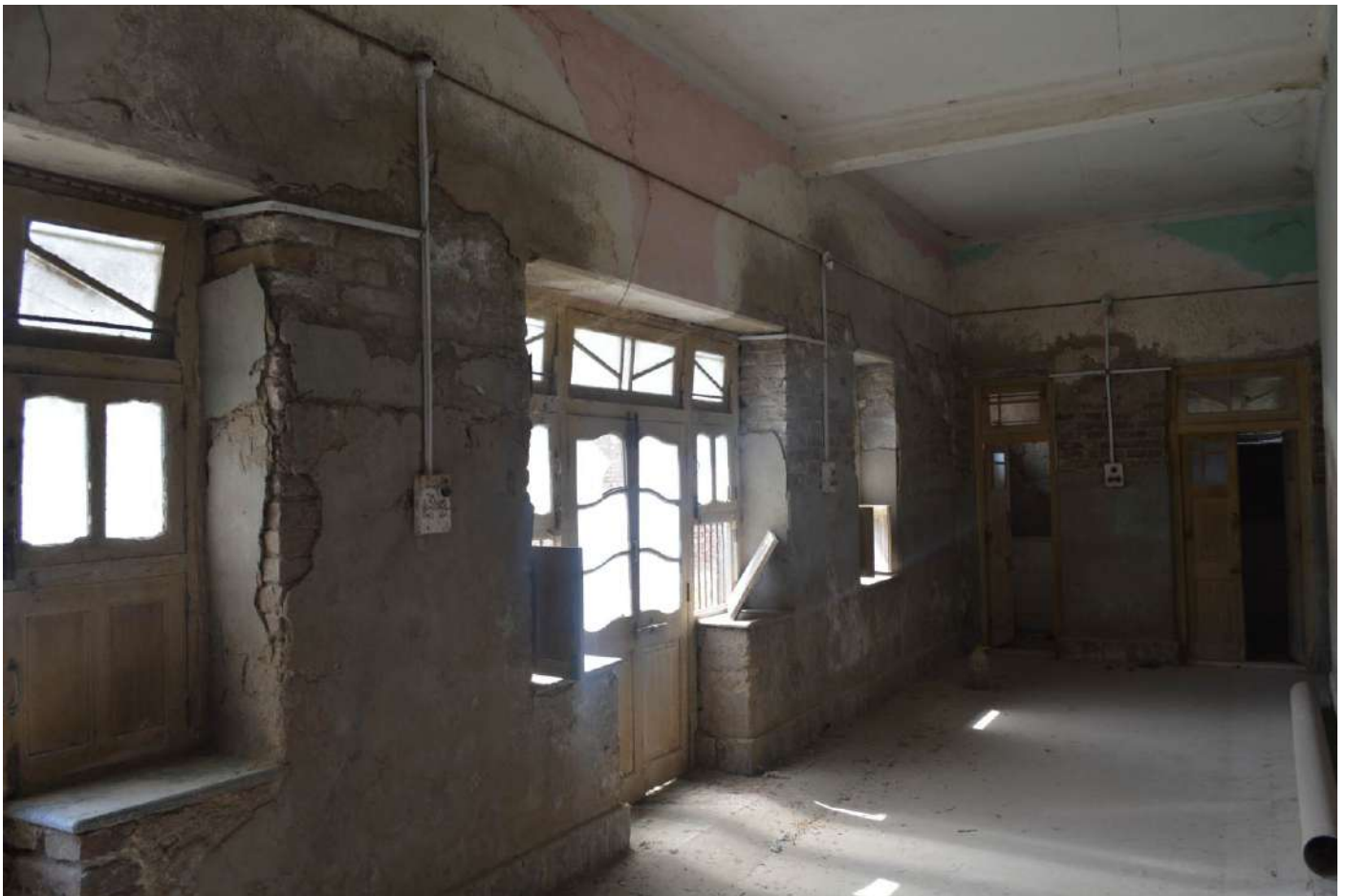
INTERIOR VIEW OF LEFT SIDE VERANDAH
