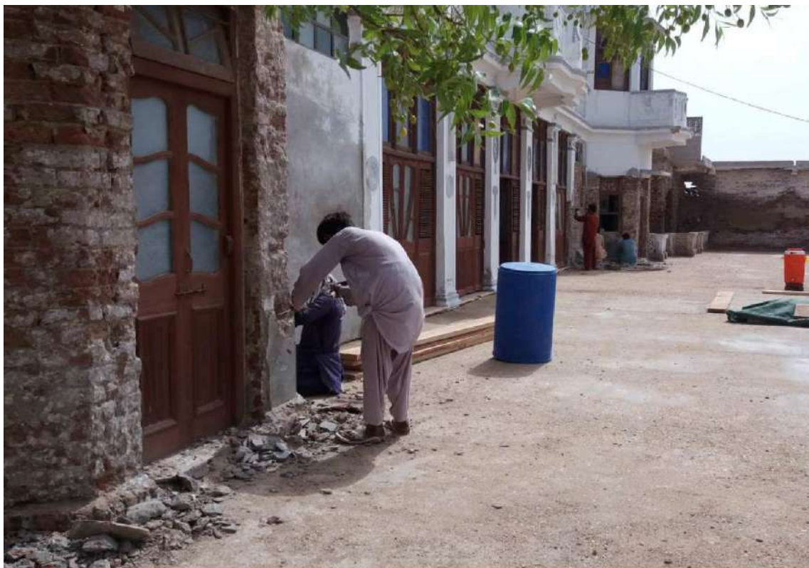
Scraping the moisture affected area of the walls
