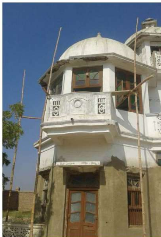
Plastering of right side of facade are in progress
