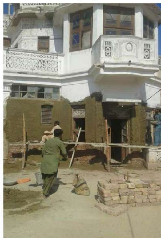
Labours are busy plastering upto lintel on the left side of facade
