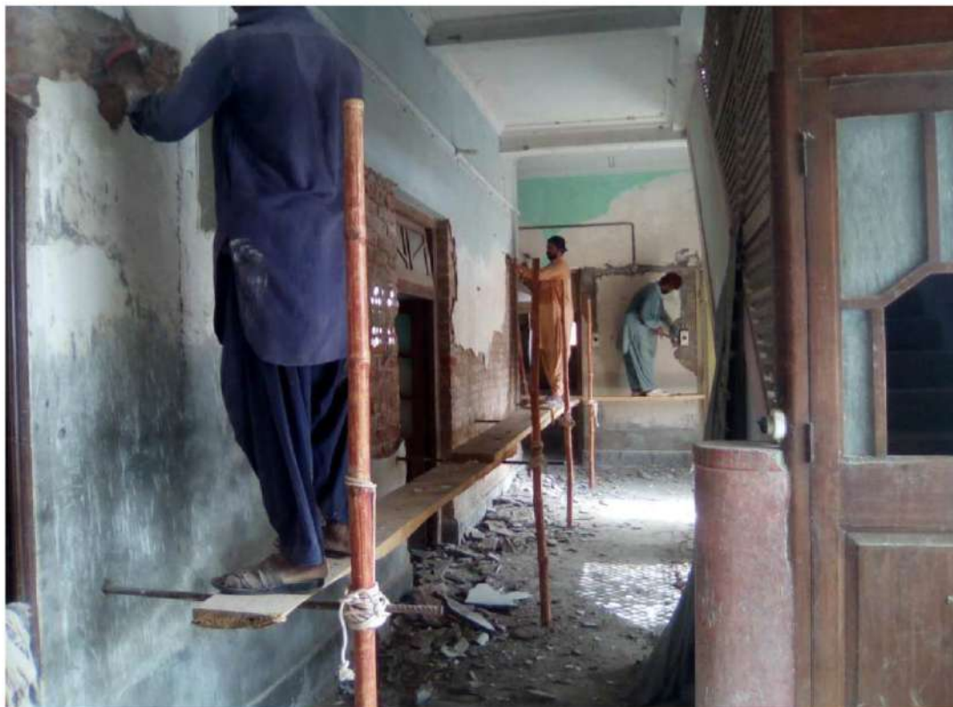
labours are working to remove the salt effected portions of walls
